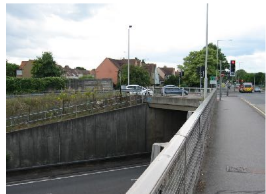
The drop from the slip road to the A2 main carriageway: 90 degrees at the walled section; probably 80 degrees on the grassed area above. Note the houses very close to the west side of the slip road.
