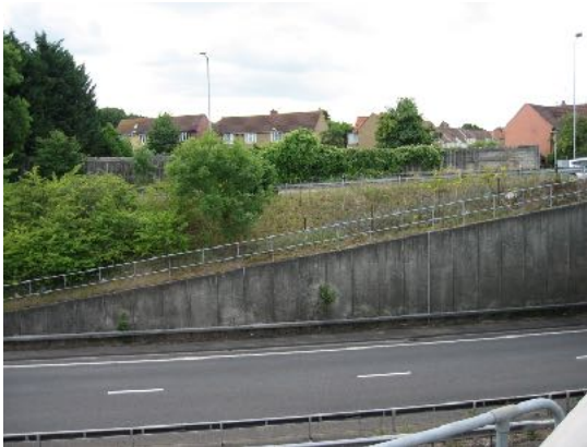
The drop from the slip road to the A2 main carriageway: 90 degrees at the walled section; probably 80 degrees on the grassed area above. Note the houses very close to the west side of the slip road.
